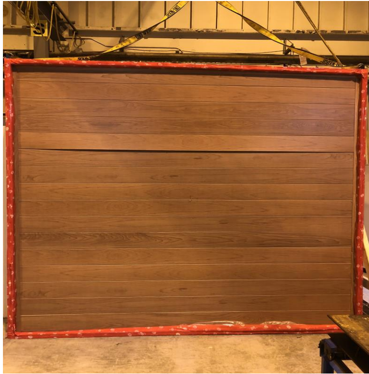
Photo 2 – Wall Section (Cladding Horizontal) post test
