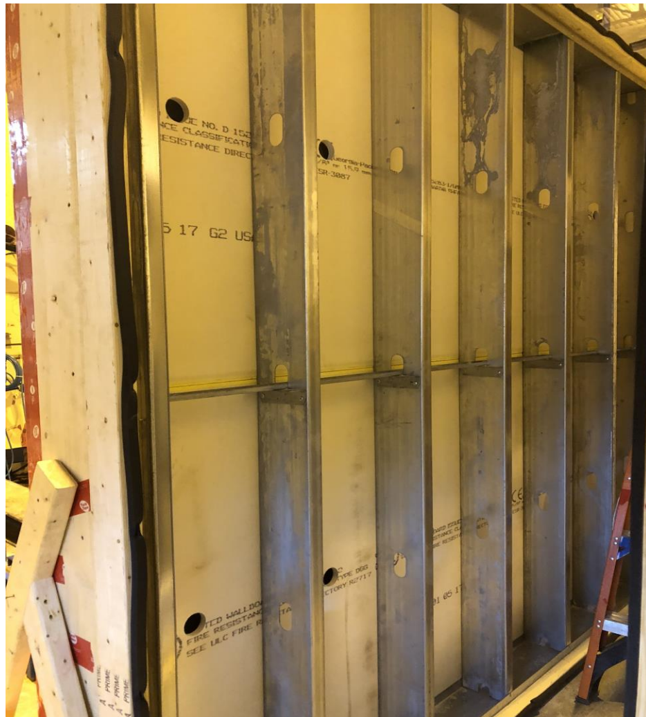
Photo 3 – Wall Section (Studs)
